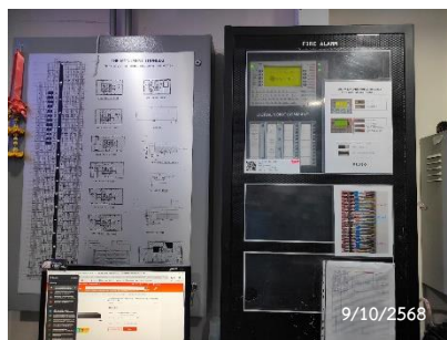
Fire Alarm Control Panel
