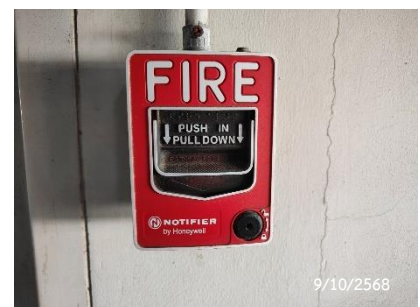
Fire Alarm Manual Station
