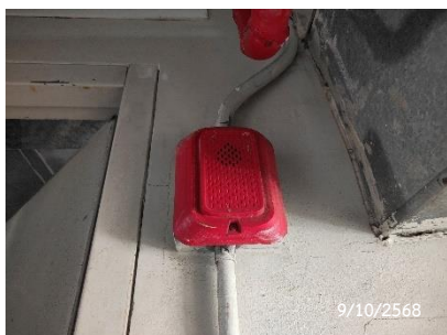
Fire Alarm Horn Strobe
